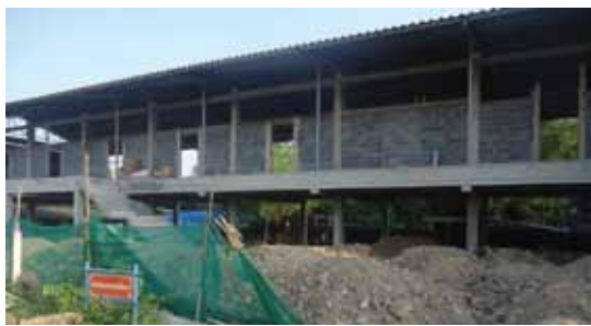
▶ Indorama Polyester Industries (Rayong) provided soil to the Community School in Mapthaphut for use in land leveling in preparation for a new school building. Over 300 m 3 of unneeded soil was moved from our plant to the school with IEAT permission.
