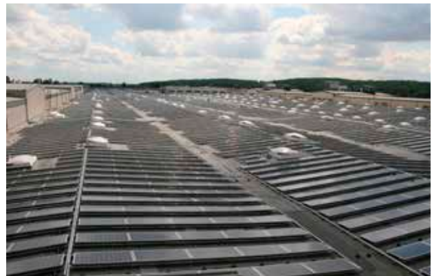
Photovoltaic panels installed at Trevira
