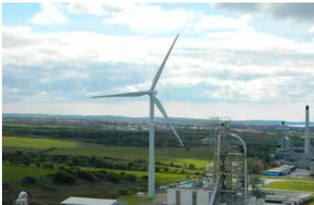
Wind generator installed at Orion Global Pet
