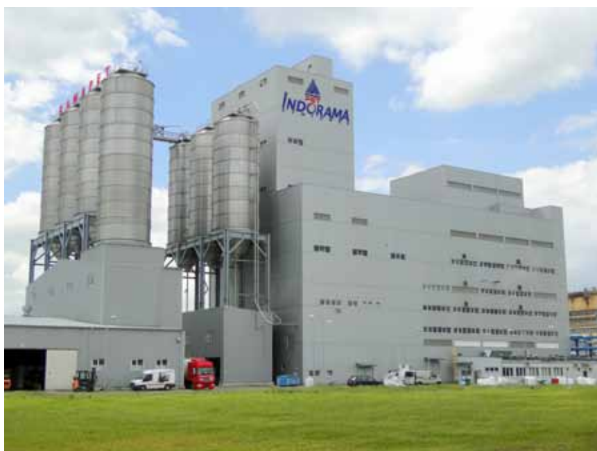
▲ Manufacturing facilities at Indorama Ventures Poland.
