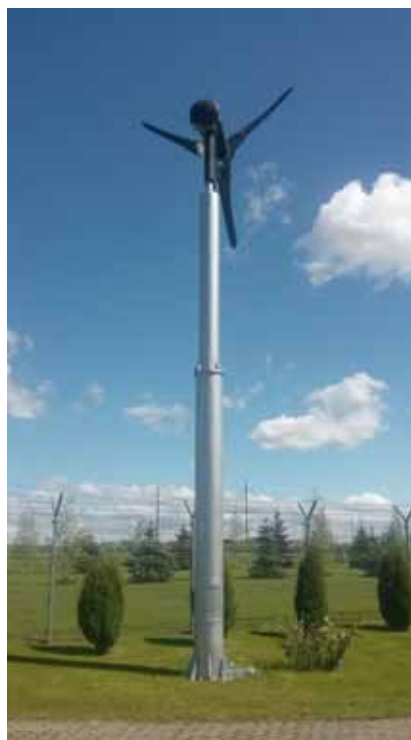
▲ Wind generator installed at Orion Global Pet, Lithuania.
