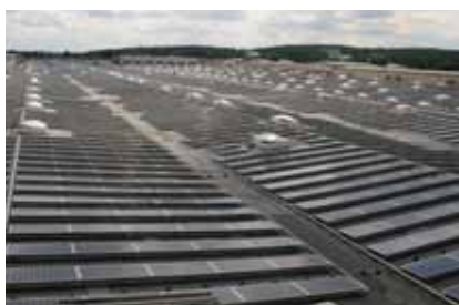
▲ Photovoltaic panels installed at Trevira, Germany.
