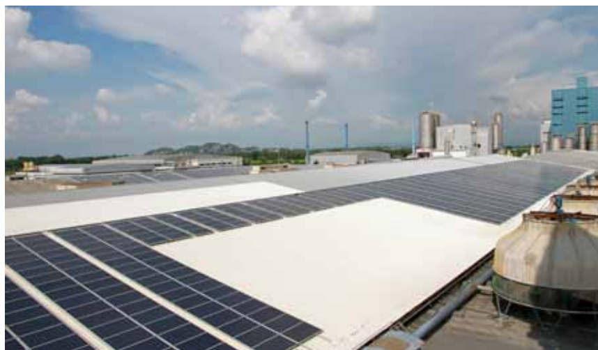
1 MW Solar Power Project at Indorama Holdings, Lopburi, Thailand. ►
