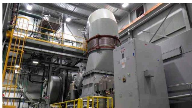
Indorama Ventures PTA Montréal (IVPTA) puts in service a turbo-generator unit that helps reduce about 20% of the electrical consumption of the company. The turbine generates on average 6,700 kW from steam, equivalent to the consumption of 2000 houses. This project allows IVPTA to be more efficient in terms of energy, to reduce our processing costs and to maintain our competitiveness in the PTA market.
